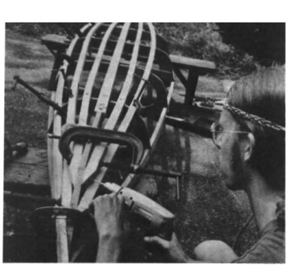
WORK from middle of craft toward ends when installing strips to prevent warpage.
